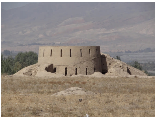
The stabilised tower
